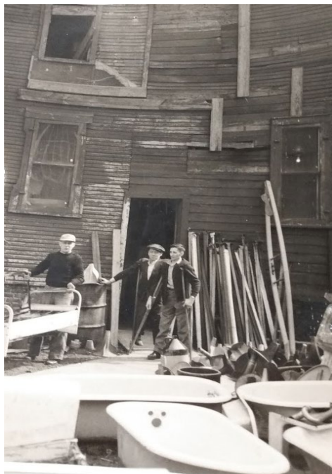
The old Bethel being demolished.
